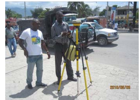
ONACA Field Work – Surveying in Port-Au-Prince
