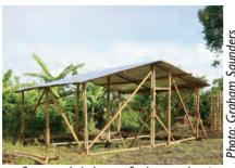
Structural skeleton of a house, showing cross-bracing
