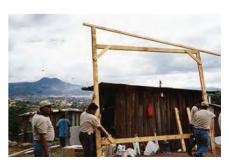
Shelter assembly using prefabricated walls
