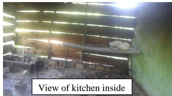
View of kitchen
