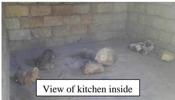
View of kitchen
