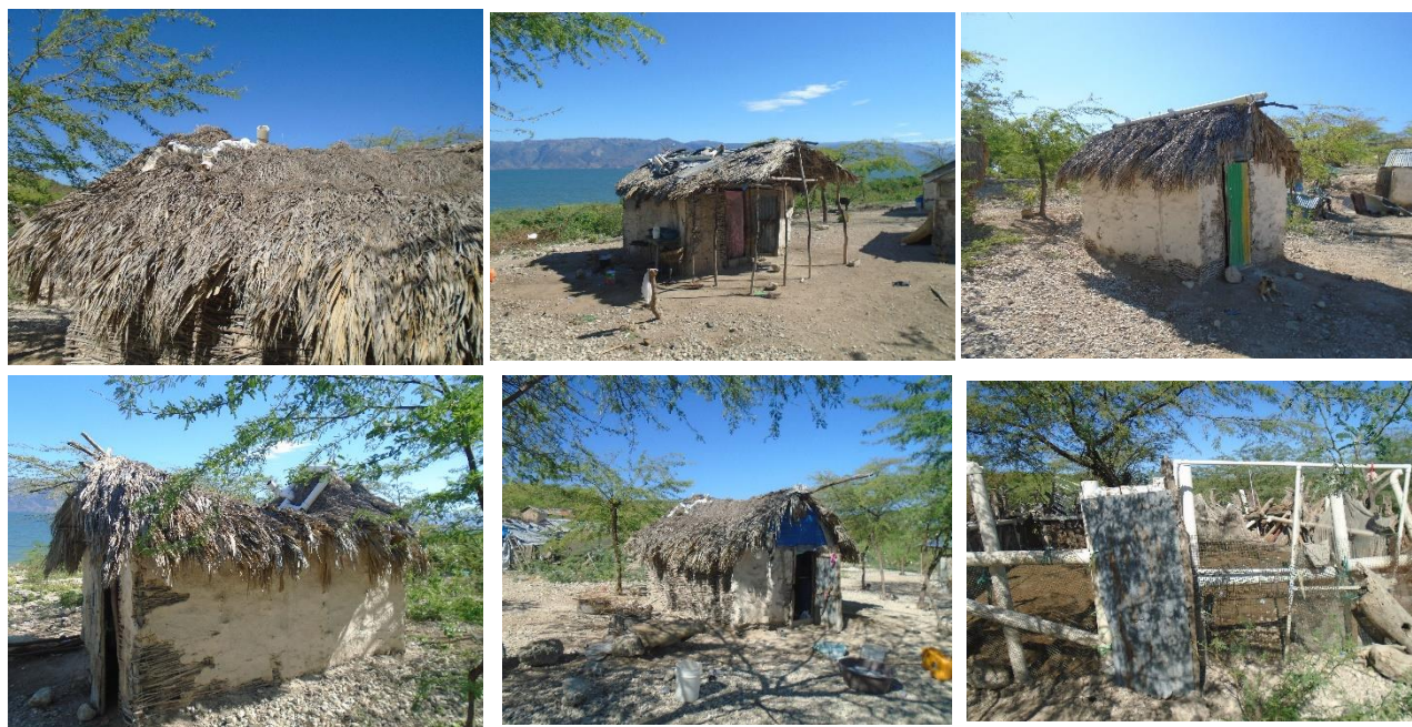
Figures F3 to F8: Remnants of CH Cages in Kanez-Belizè (specifically Madam Belizè), Used to Hold Down Thatch Roofs and as a Goat Corral
