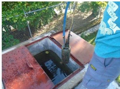
Figure F45: Filter that has not worked in over 1 year, at Lake Peligre Hatchery.
