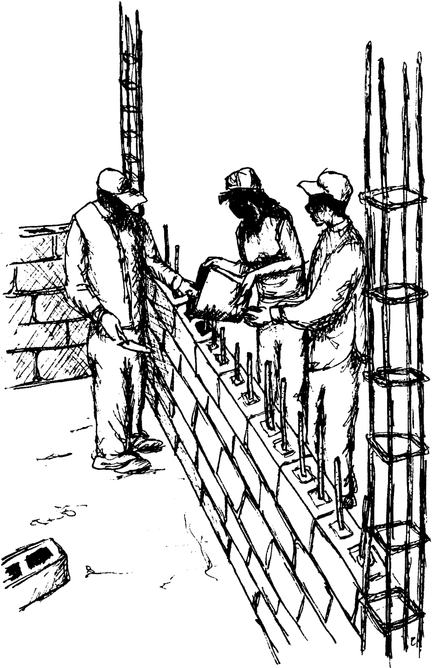
Figure 7-24. Concrete Block Installed over Vertical Rebar. Workers Are Filling Hollow Cores with Grout to Create a Reinforced Concrete Block Wall.
