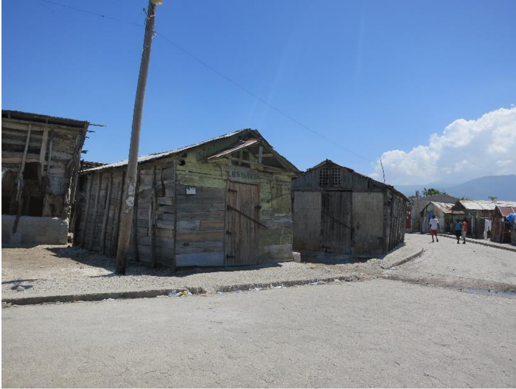
Figure 13 Houses in Cité Soleil (Joos, September 2013)
