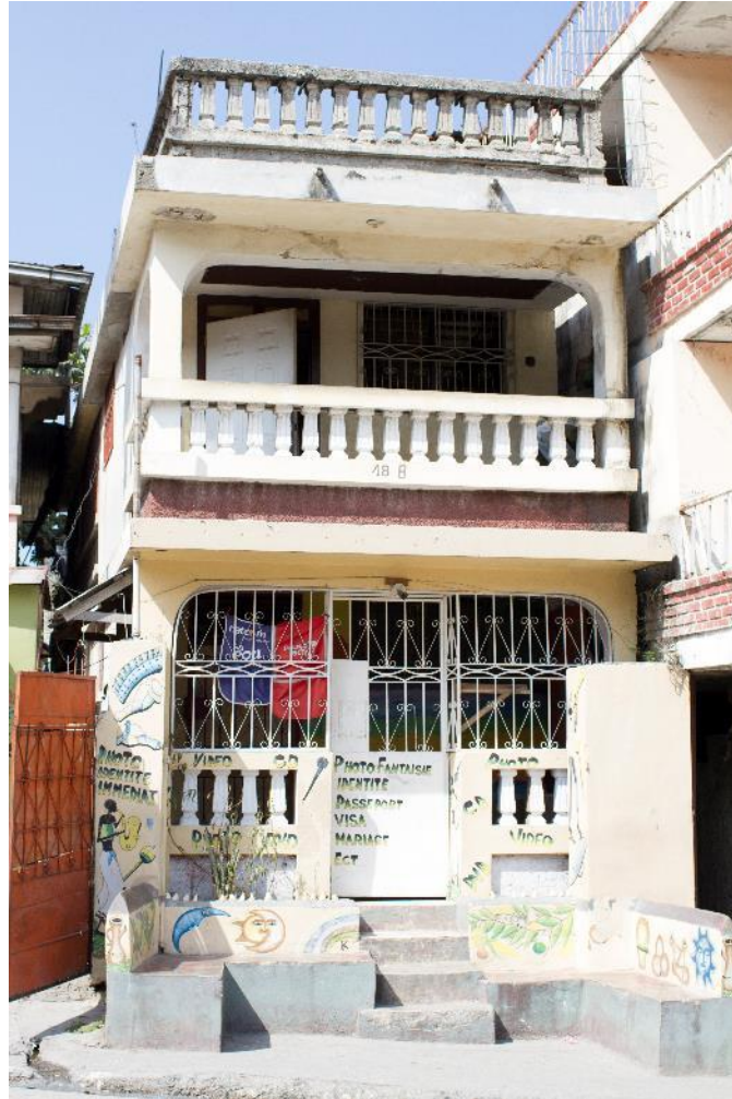
Figure 40 An apartment building in Bolosse 4
