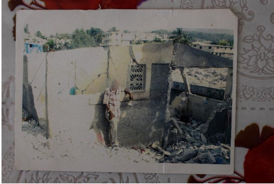
Figure 15 Photo of G. Defils standing in his collapsed apartment, 2011
