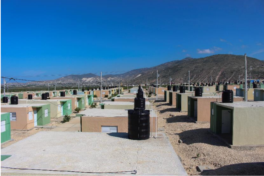
Figure 14 View from the rooftop of G. Defils (Joos, May 2014)
