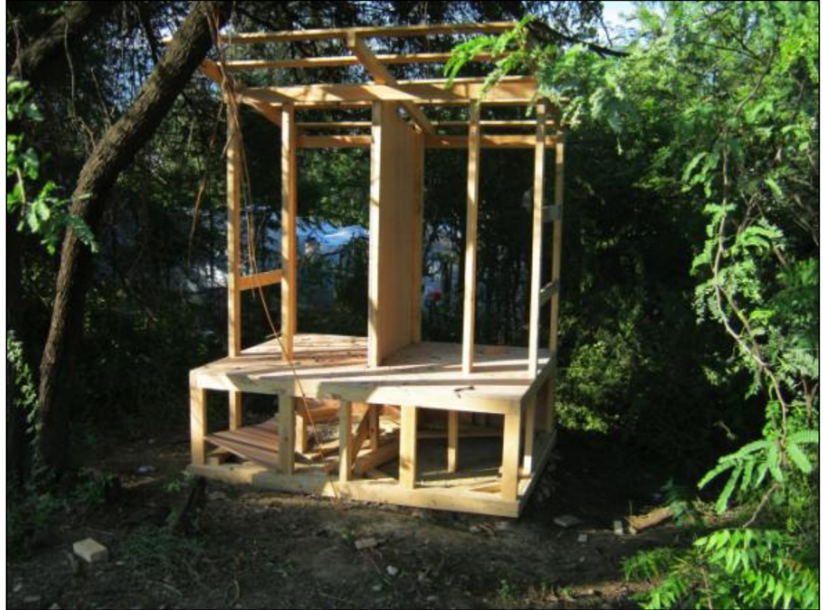
PHOTO T10: Wooden Structure
