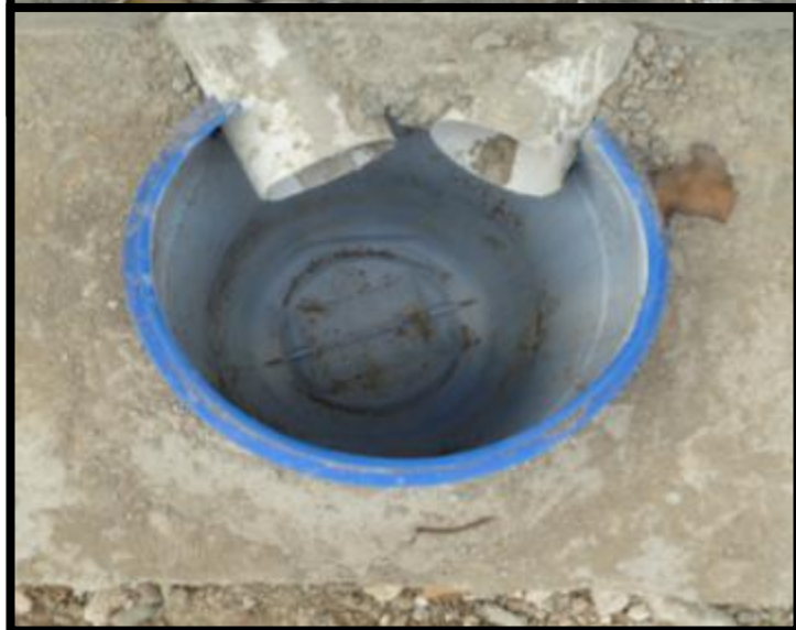
Photo K108: Leachate drain from 2 compost compartments collected in a single 15 gallon drum
