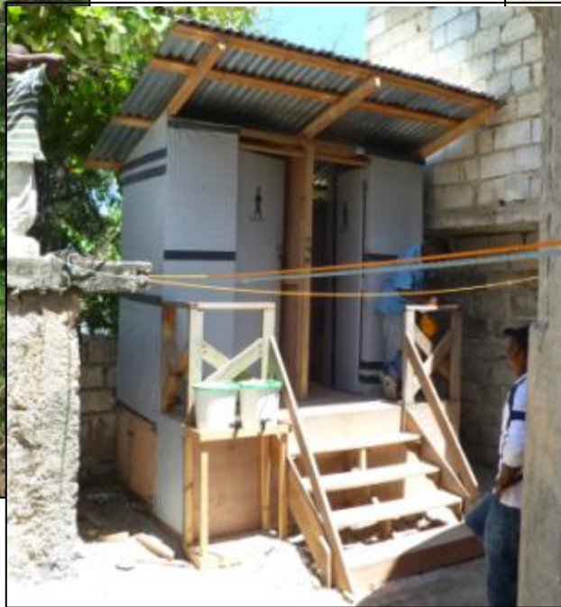
PHOTO T16b: GOOD positioning of SOIL UD toilet with just enough space for chamber access
