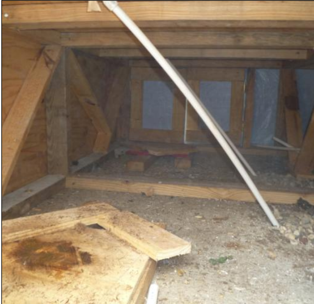
PHOTO T1: Chamber beneath toilet
