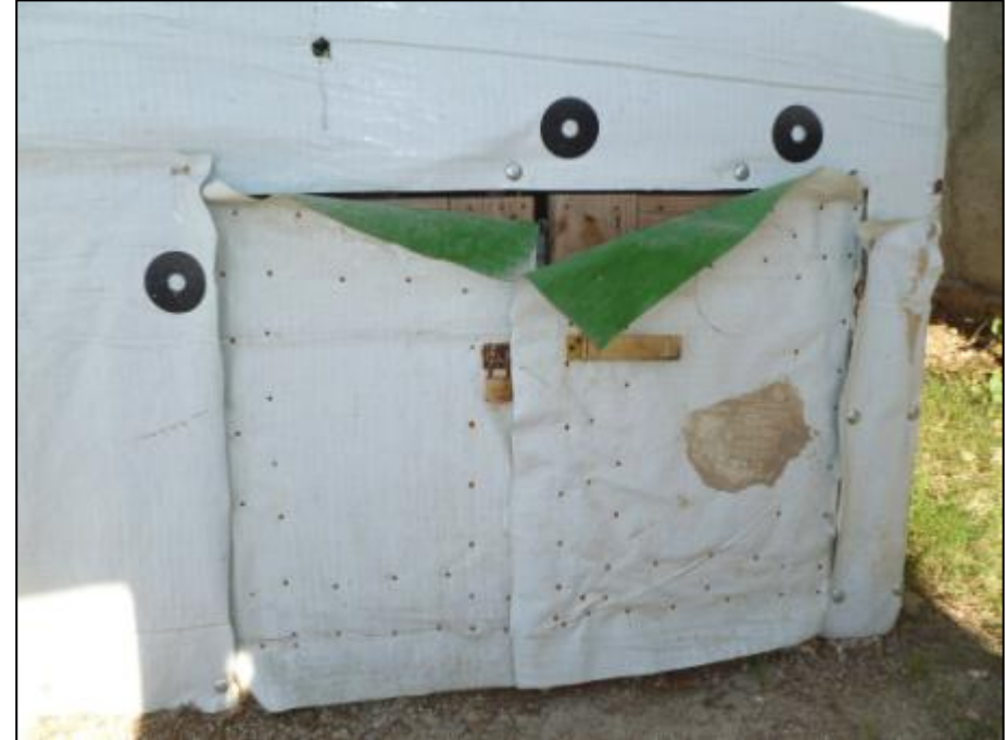
PHOTO T12: Close-up on chamber doors
