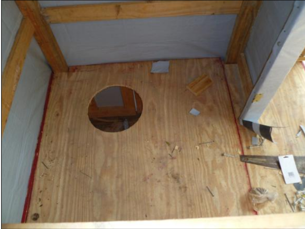
PHOTO T5: Poophole cut in plywood floor
