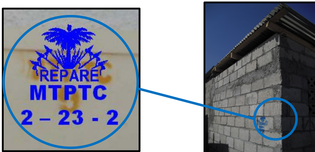
Fig. 12 – Example MTPTC Stamp of Repaired House
