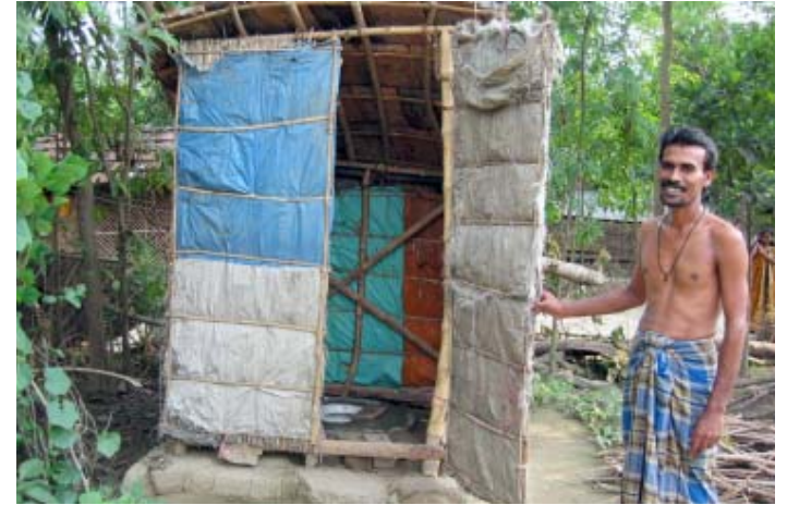
ABOVE Use of bamboo and plastics in making the super structure while the sub structure is strong and perfect. Vidyasagar colony, Kalyani, West Bengal India.
