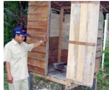
ABOVE Raised platform of a toilet to avoid seasonal flooding in Indonesia.
