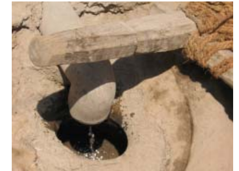
ABOVE AND LEFT A local community innovated this unique way of absorbing the wash-waste water from a wash room in to a perforated and buried earthen pot filled with pebbles and stones in a village in Maharashtra state in India. This kept the road dry and clean which used to be muddy and dirty before.
