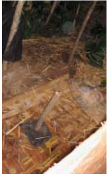
LEFT A direct pit latrine constructed immediately after triggering of CLTS in Uletana Bakole village near Arbaminch in Ethiopia. Notice the use of bamboo, mats and plastic which are locally available materials in construction. Often latrines are gradually improved.
