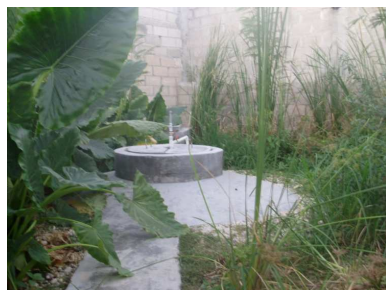
Biogas Unit or Biodigester
